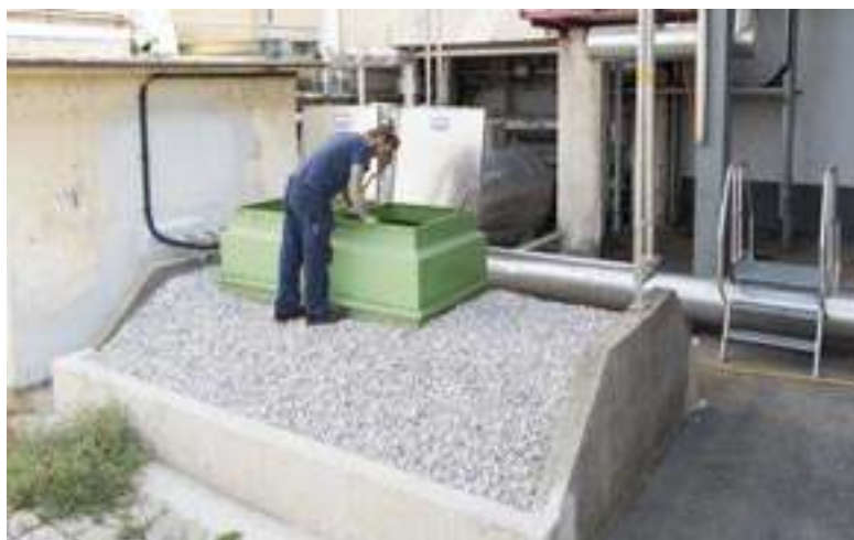
Harald Stassler inspects a manhole shaft (underground solvent tank)
