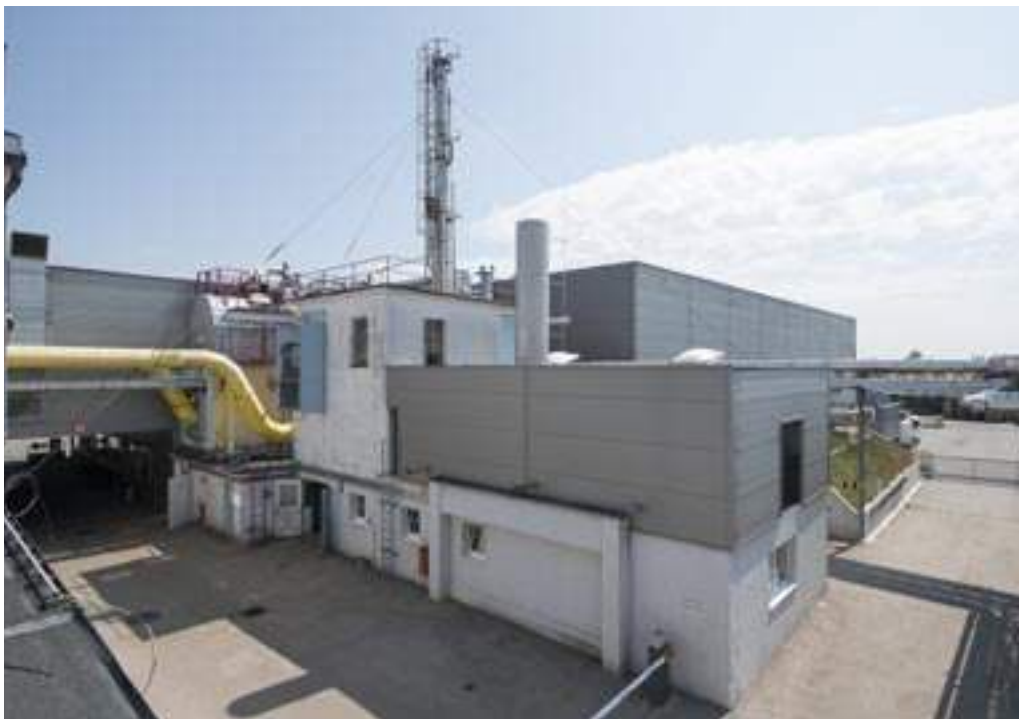
View of the solvent recovery plant
